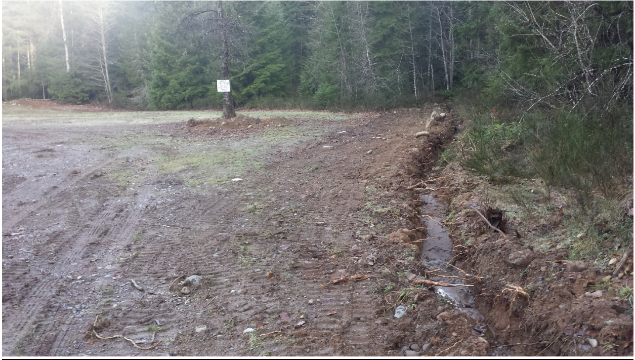
December 2014, Ditching to prevent roadway water from flooding site
