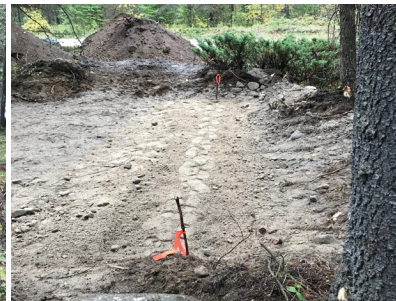
FINAL SITE-PREP LEVELLING
